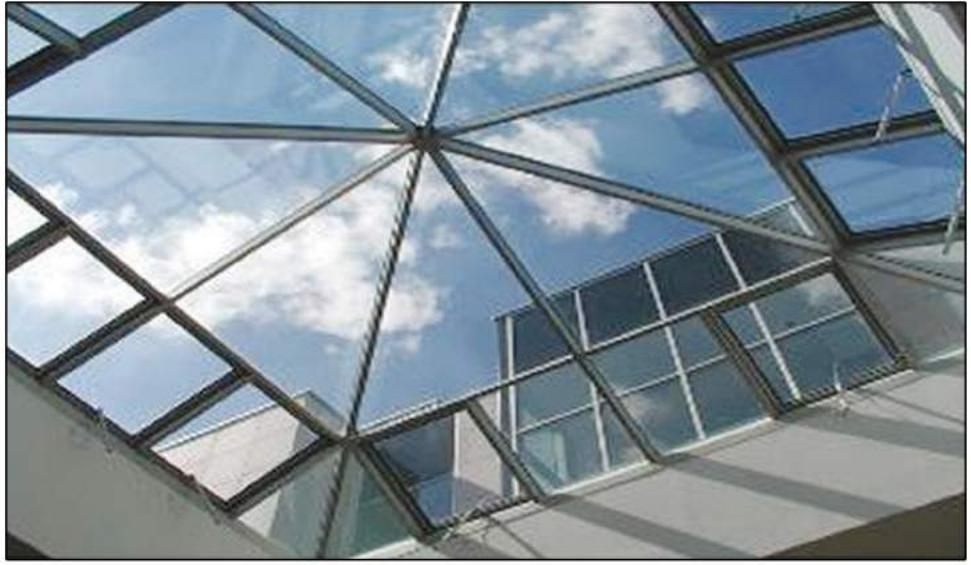
Skylights can be implemented by using special aluminum sections with high thickness fit all the required sizes, tempered glass, and heat-treated glass of different normal and reflective colors. In addition, they can be implemented by using stained glass, Alixan panels, or Decosan panels according to high professionalism which ensure full insulation of water and dust.
